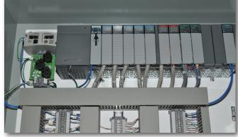
PLC control panels utilize the Allen Bradley PLC family and can be either the SLC or Control Logix package. All controls are pre-wired and tested at the factory. All systems include remote programming capabilities.
