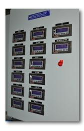
The weighing system includes load cells, summing junction box, digital weight indicator (or direct PLC scale card), and communication module to PLC. All scales are NTEP approved and are fully tested with certified test weights. Automatic calibration cycles are available as an option, as well as automatic test weigh application to verify scale accuracy at the touch of a button.
